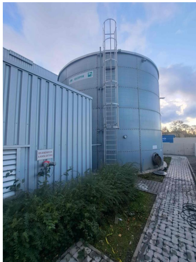
Te inspecteren tank
