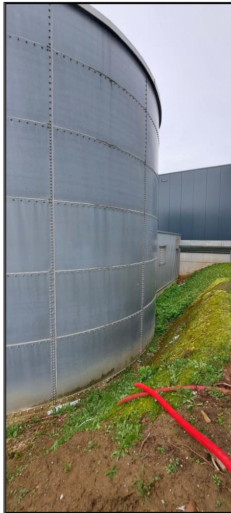
Te inspecteren tank
